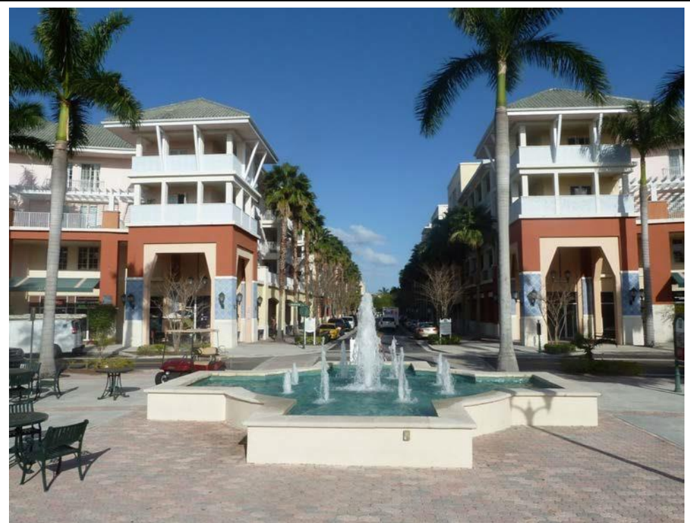
Well-designed town centers can provide gathering places for communities and the location for restaurants and neighborhood-serving retail as well as larger regional destination retail. In an urban format, parking decks can be shielded from roadways and pedestrian spaces, with active uses lining the front façade of garages to soften their physical and visual impact.
