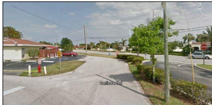
ABOVE-LEFT: Interior roadways throughout the proposed CRA are without sidewalks, lighting, and curb and gutter infrastructure, which reduces access and creates safety hazards for pedestrians and cyclists.
