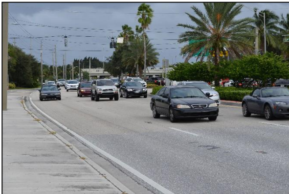
ABOVE-LEFT: Forest Hill Boulevard is a six-lane arterial carrying more than 43,000 cars daily. The roadway was constructed with minimal sidewalks and no bicycle facilities, and its configuration leaves no room for these amenities to be added or modernized to meet current market trends for improved multi-modal function or a Complete Streets network.
