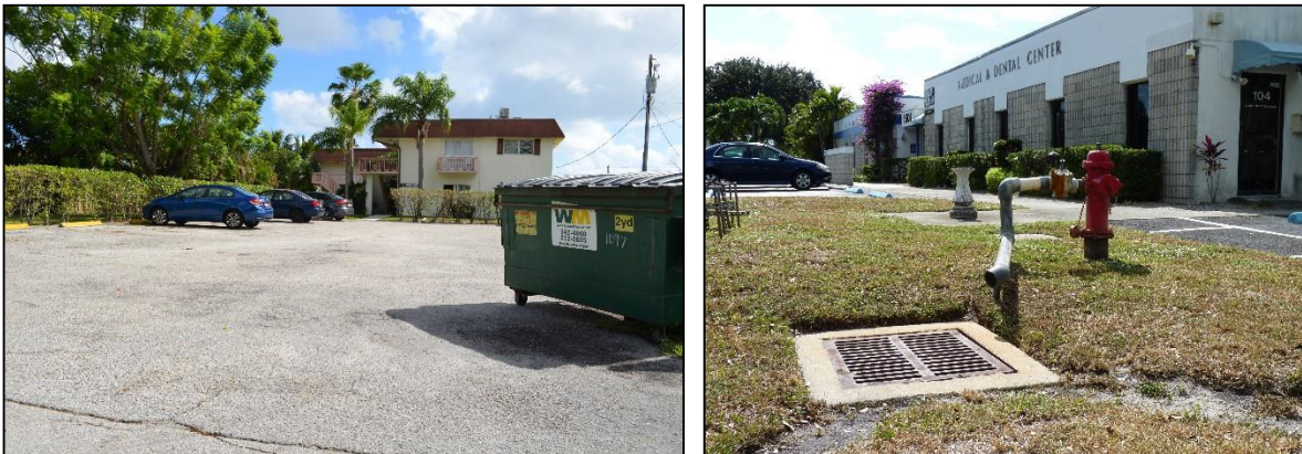
Poor property maintenance and deficient property conditions are a reflection of the declining assessed values in the CRA.
